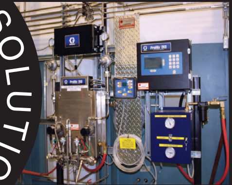
2K Finishing Solutions
